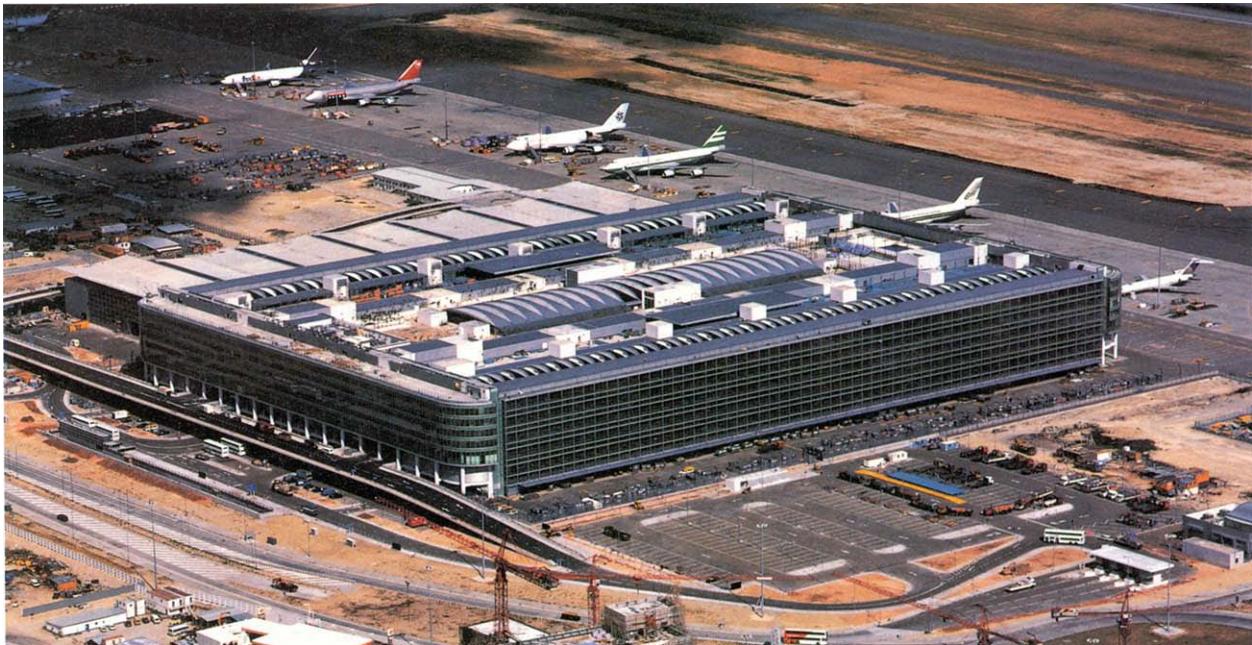
Image 1: Hong Kong Air Cargo Facility (HACTL)
