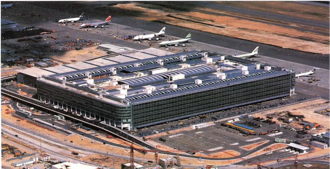
Image 1: Hong Kong Air Cargo Facility (HACTL)
