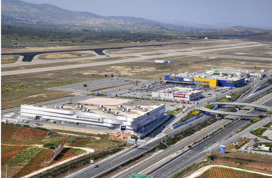
Athens Airport Retail Park hosts factory outlets and mega-stores.
